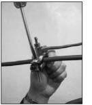
**12.** Tap into the water supply line using the saddle valve provided. Follow the directions on the saddle valve bag.
